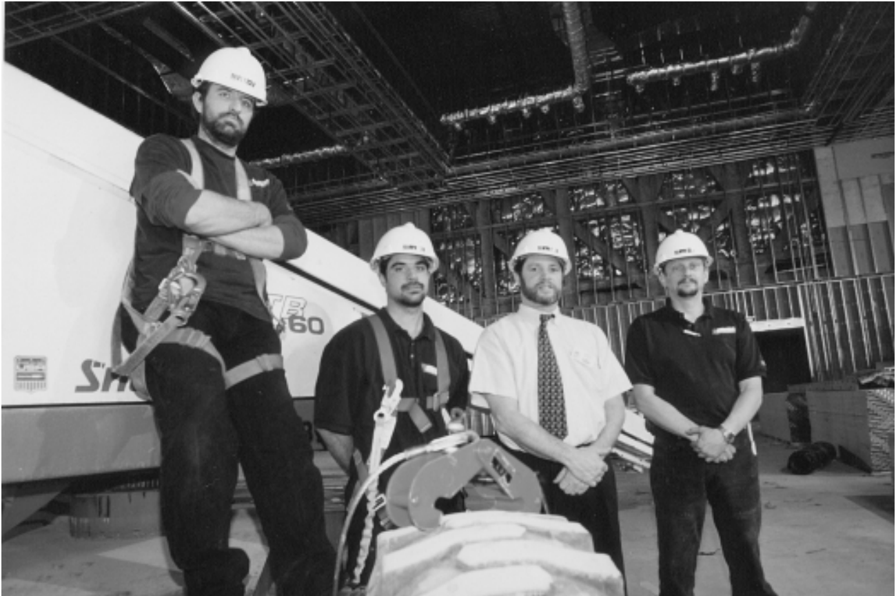
Rigging in the new ballroom, the MSI crew is Donald Ethridge, Paul Magellan, Gary McIntyre, and Pat Borovicka.
